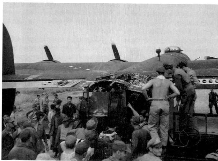
Battle Damage, Members of the 484th Bomb Group gather around an olive drab B-24 that has suffered damage to the tail turret, killing the tail gunner. Notice the right elevator was completely shot away, and the left elevator was hit also.
