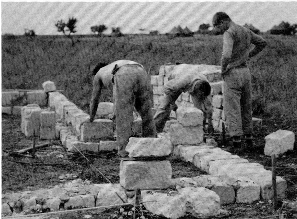
Building a "Tufi Block" house at Torretta.(10-1)
