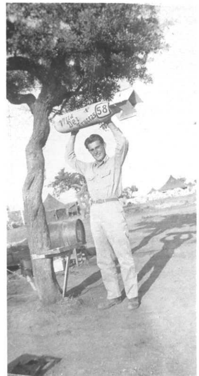
Charles Walling, 826 Squadron area
