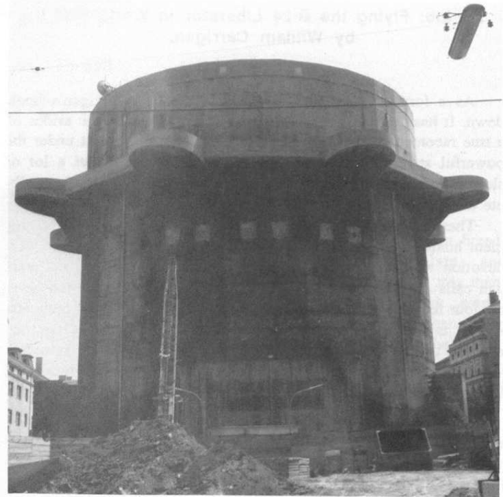
Flak tower in Vienna near the Slifln Barracks. It was called the "Sliflnbunker." It was equipped with double mount 12.8 CM cannons on top of the main platform and 2.7CM and 3.7CM cannons mounted on the outer ring of the tower.
