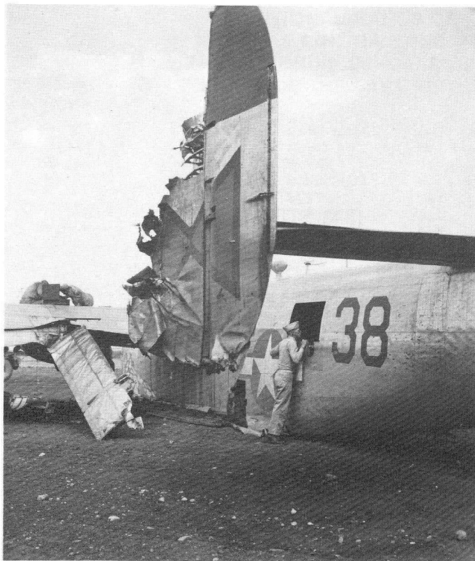
Ship #38 825 Squadron, sustaining heavy battle damage manages to make it back to the base at Torretta. It appears much of the destruction took place when she bellied in as parts were flying through the air. Notice the inboard section of landing flap hanging by only one hinge. The laws of the air were lopsided, some aircraft sustaining major damage would maintain flight while others seemingly unscratched were seen dropping out of formation never to be seen again. Robert A Harrison photo 825 Sq.
