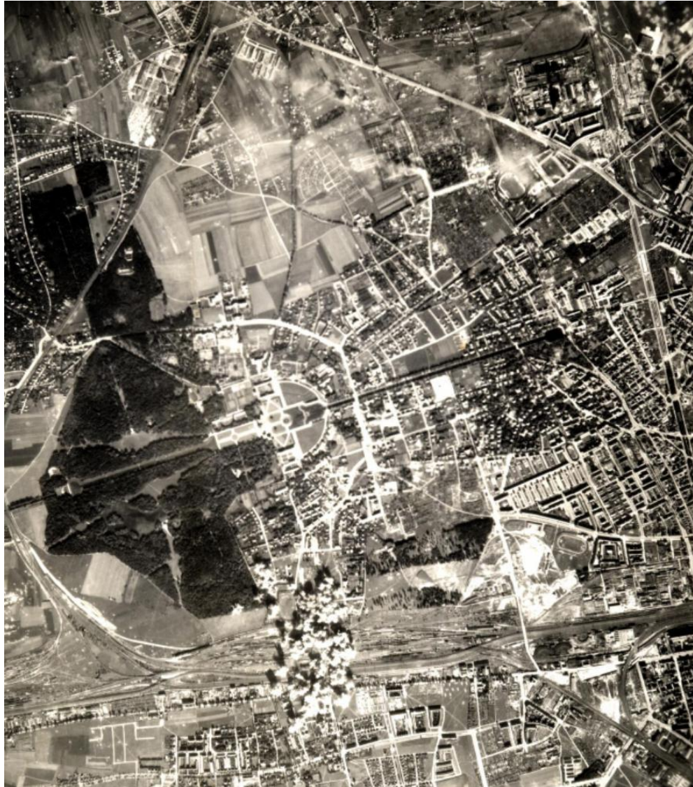
Munich West Marshalling Yard, Germany from a ship Oct. 4, 1944
