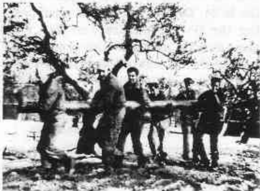
Stealing pipe for tent heaters!
